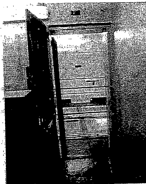
Fig. 5-19 View from inside a typical 'A wing' cell with a grille door and a solid door. There is a rebate to house the grille door in the closed position. (CM 1997)
