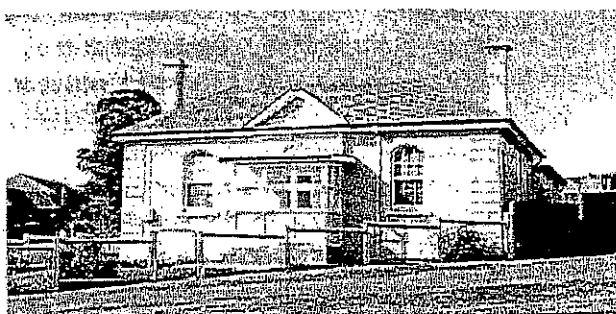
Fig. 5-35 The Police Lock-up in 1969. Note the corrugated iron roof which is currently concrete tiled. (DPWS Plan Room)
