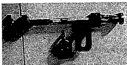
Fig. 7-11 Typical cell door bolt and lock. This lock is one of the more recent Abloy Lock types. (CM 1997)
